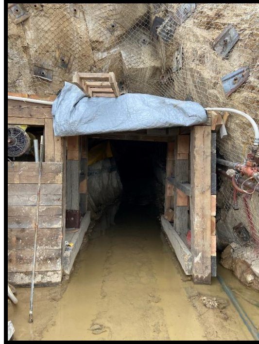
Addition of air handling equipment
