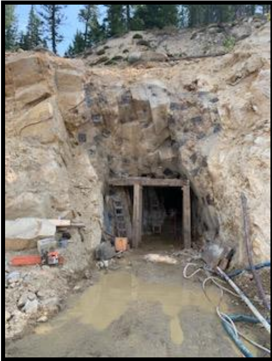
Lucky Ben Adit under Construction
