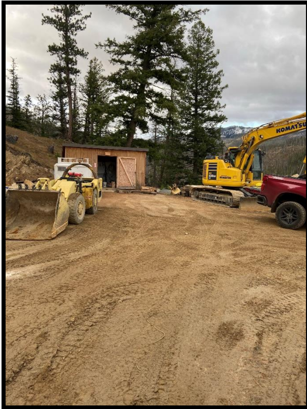
Improvements to the Lucky Ben Adit Area
